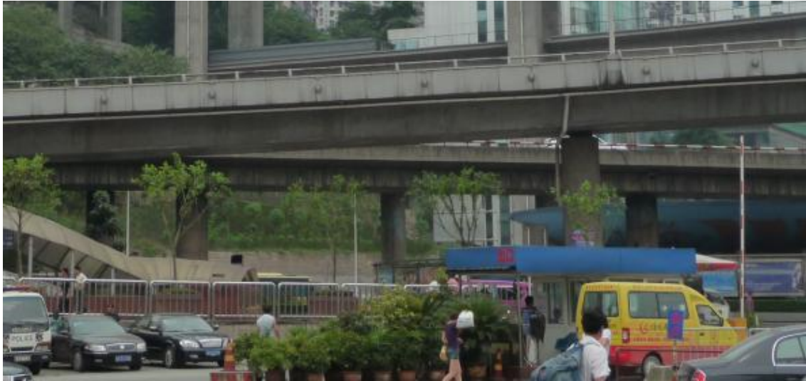
Picture 4 Pier of Original Caiyuanba Interchange
