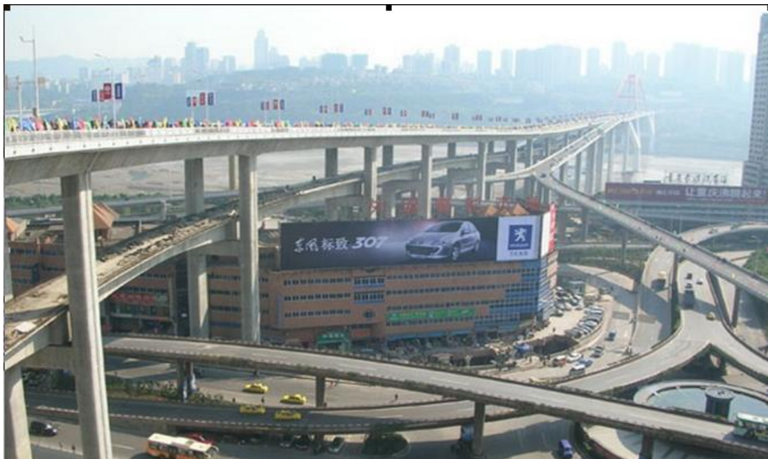
Picture 2 Caiyuanba Multi-layer Semi-directional Partial Interchange
