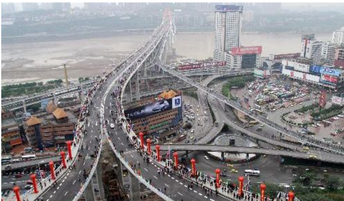
Picture 1 Caiyuanba Interchange
