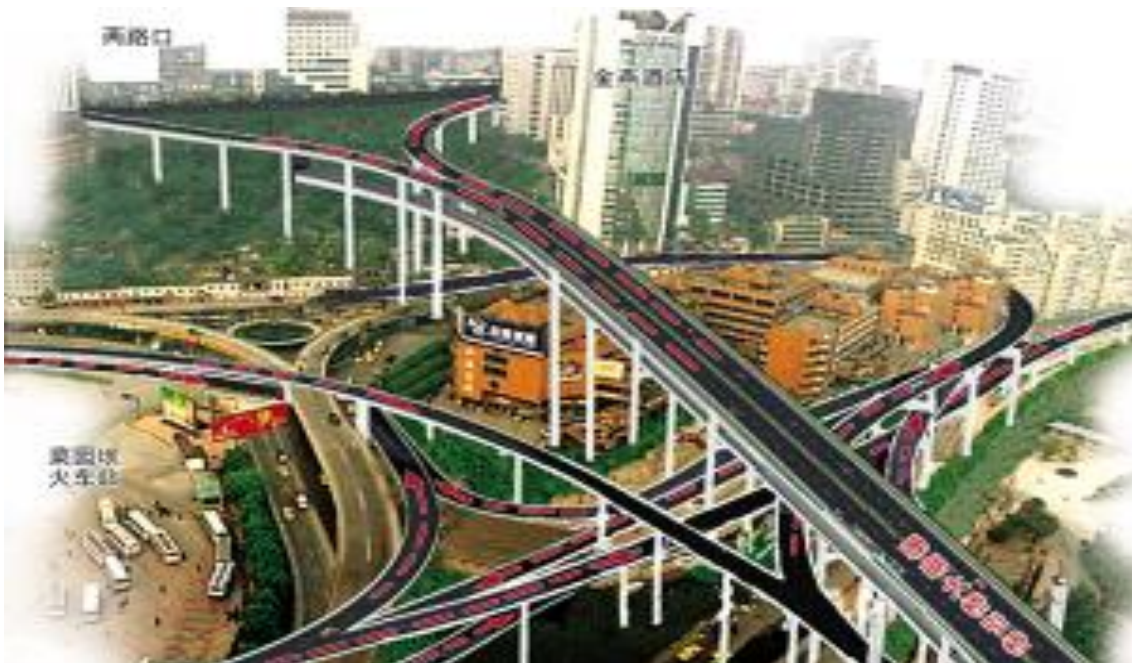
Picture 3 Multi-layer Semi-directional Partial Interchange
